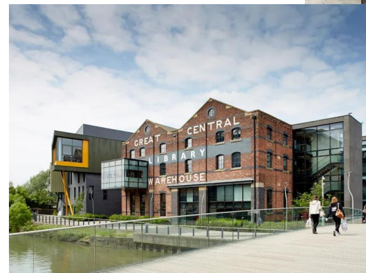
Great Central Warehouse Library
